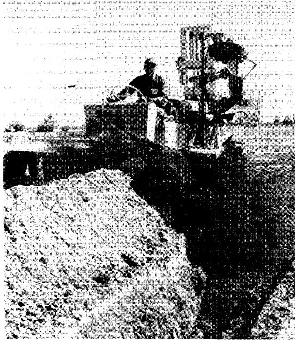
Backfilling with machinery
