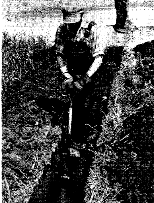
Trenching with a spade
