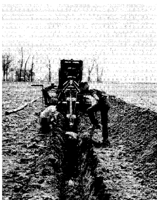
Blinding drain with a spade
