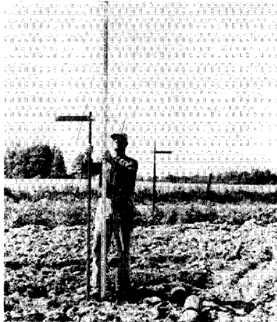
Setting targets for a trenching machine
